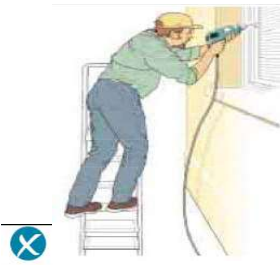
Incorrect – steps side on to work activity
